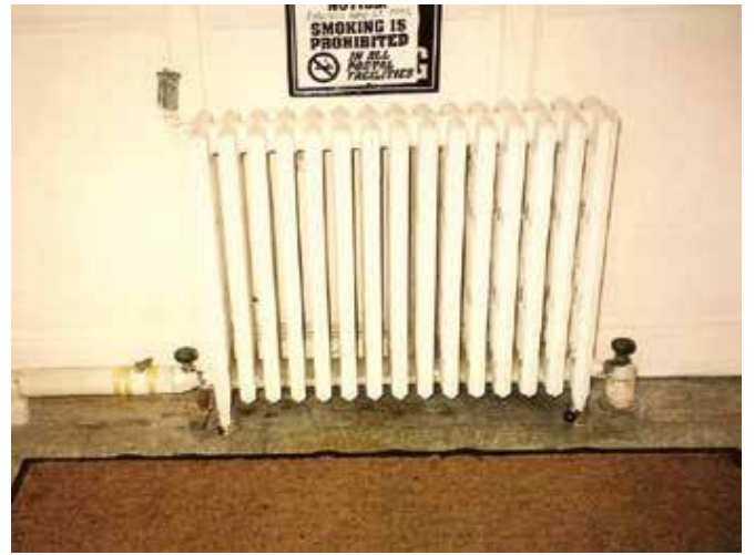
Radiator (insulation on piping and valves)
