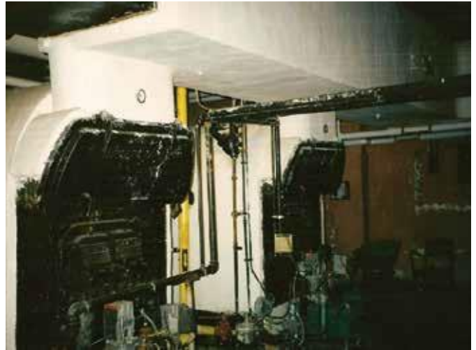
Boiler and Pipe Insulation
