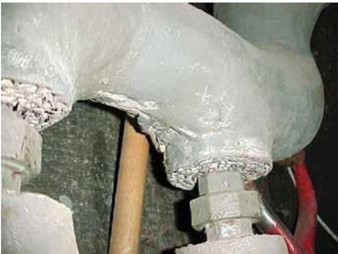
Pipe Fittings (air-cell and mud-plaster type coating)
