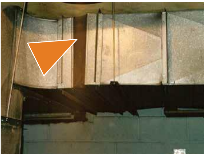
HVAC Vibration Damper (boot fabric)
