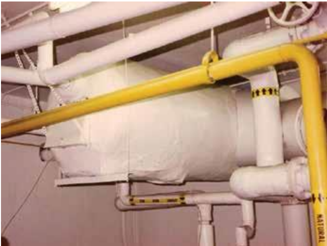
Tank Insulation
