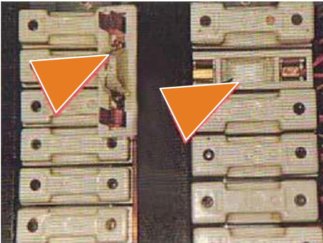
Asbestos Rope (electrical fuse board)
