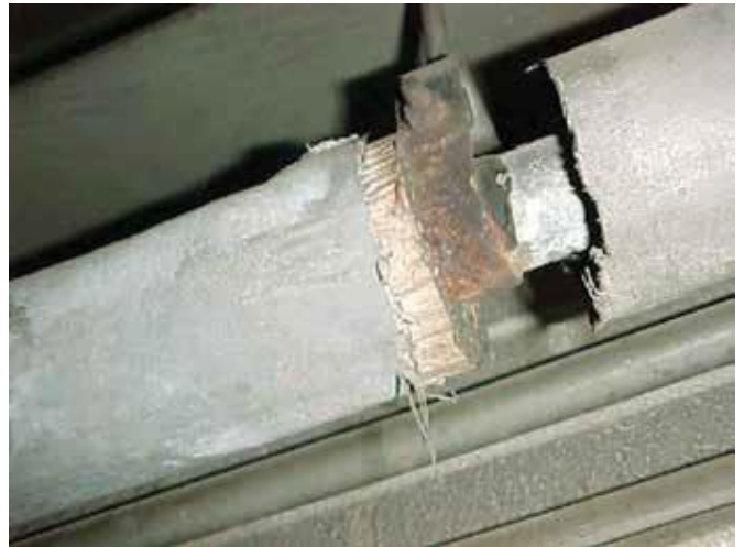
Pipe Insulation (damaged)
