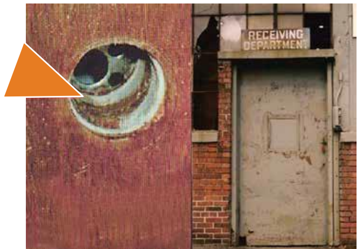
Fire Door (insulation inside door)
