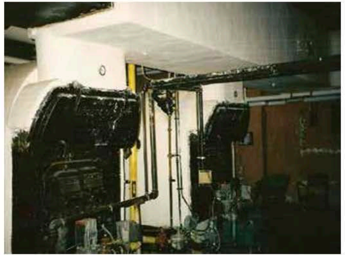
Boiler and Pipe Insulation
