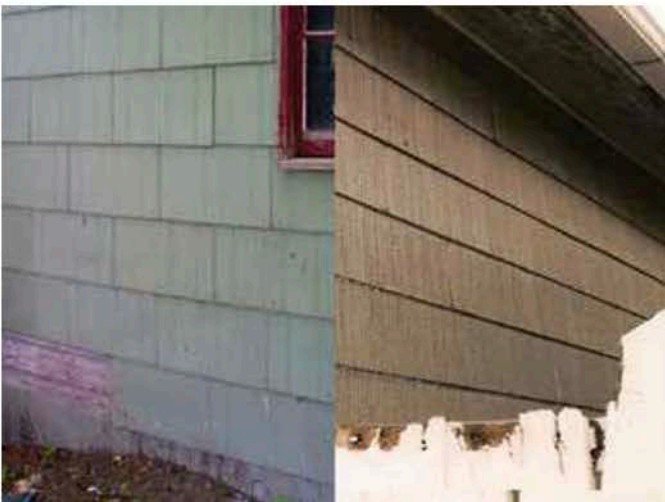
Transite Siding/Shingle
