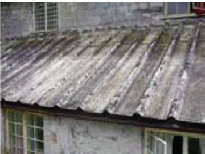
Transite Roofing (cement)
