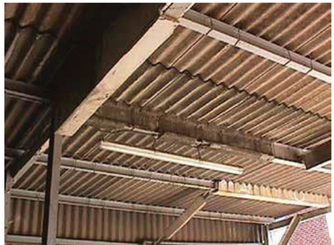
Corrugated Transite Roofing (cement board)
