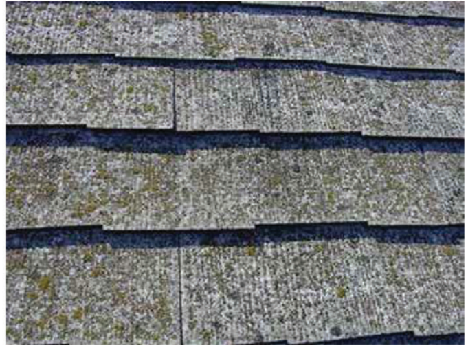
Transite Roofing Shingles
