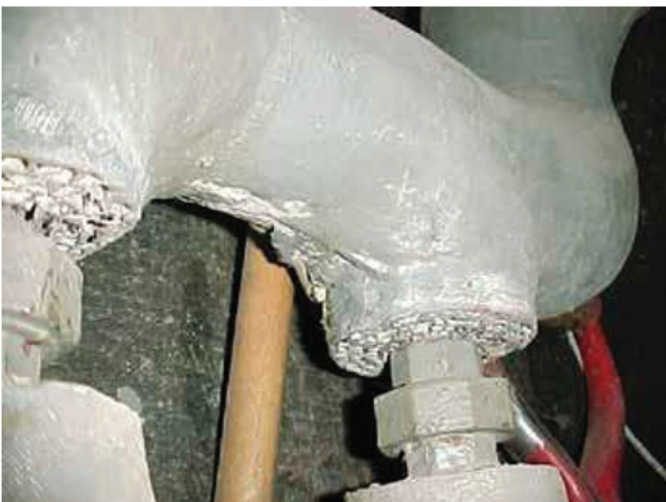
Pipe Fittings (air-cell and mud-plaster type coating)
