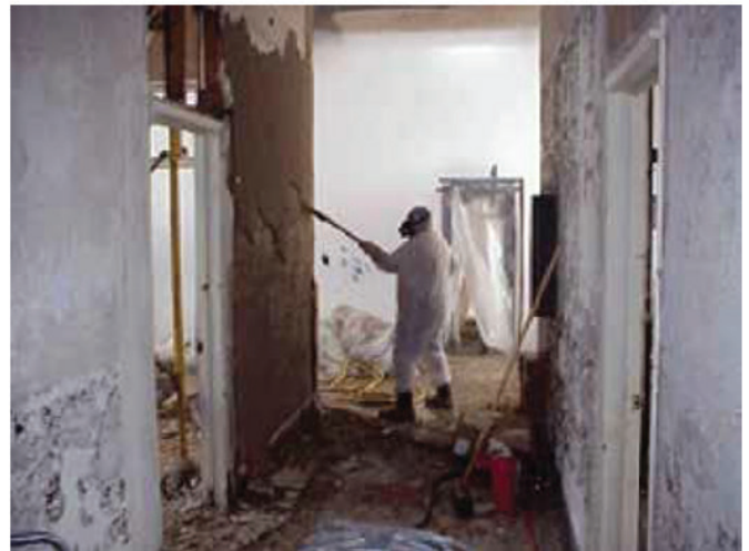
Plaster Walls (being removed)
