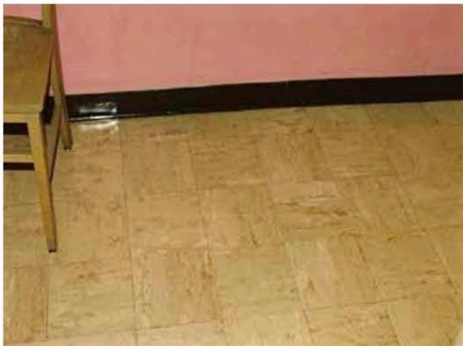
Vinyl Floor Tiles and Cove Base (most 9"x 9" and 12"x 12" floor tiles)
