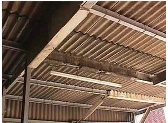
Corrugated Transite Roofing (cement board)
