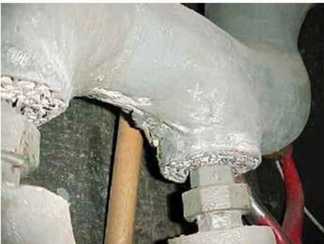
Pipe Fittings (air-cell and mud-plaster type coating)
