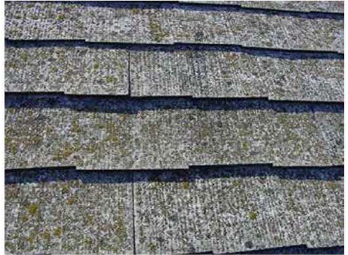
Transite Roofing Shingles
