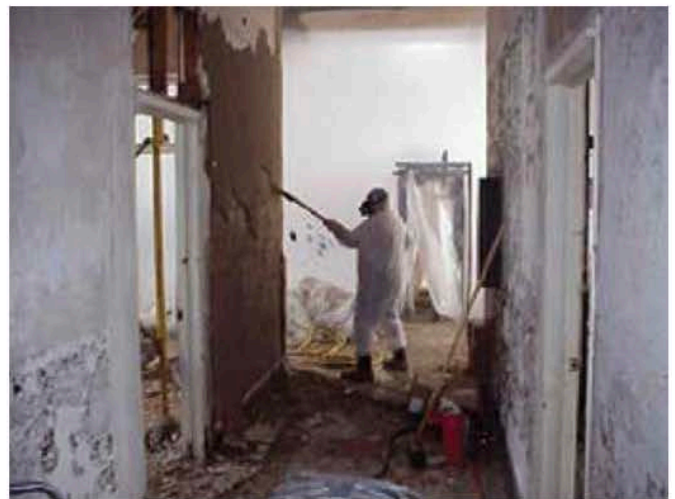
Plaster Walls (being removed)
